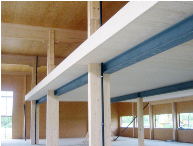
Gallery with 1t payload per m2
