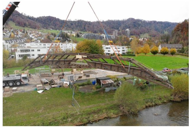
Assembly work on the bridge
