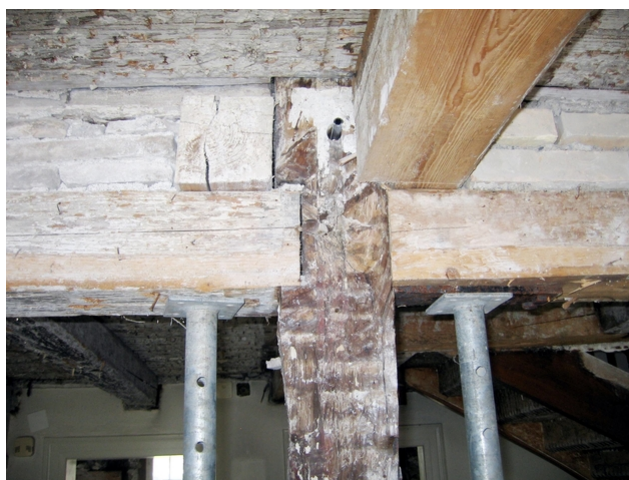
Support for beams on the first floor before renovation
