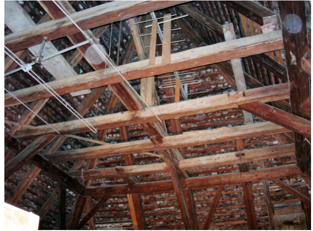
Attic before renovation
