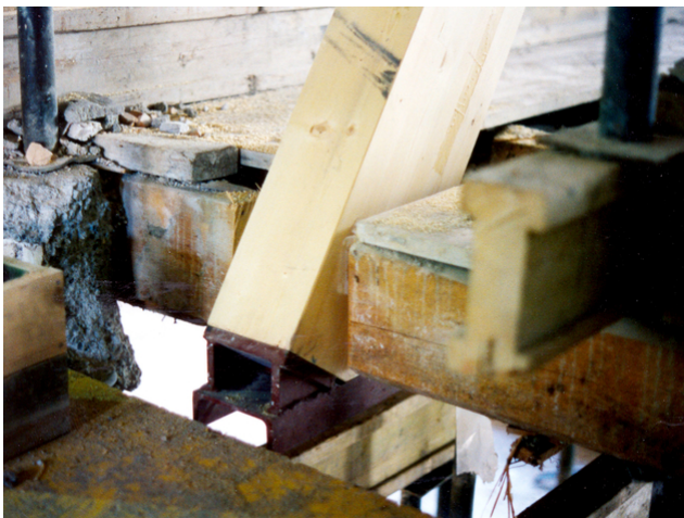
UNP beam, end support truss
