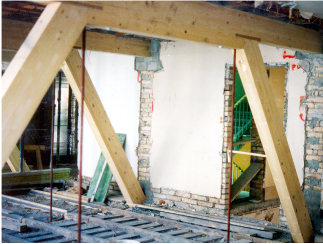
Storage in the wall
