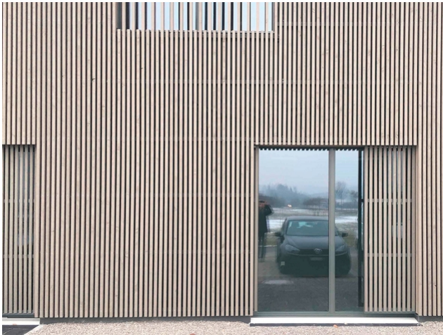
Polo Park factory building: wooden formwork facade
