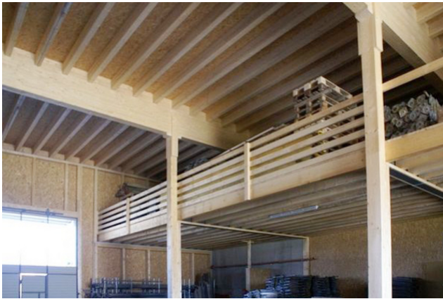
Storage space in the gallery area
