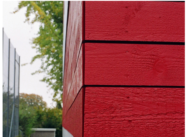
Formwork corner area
