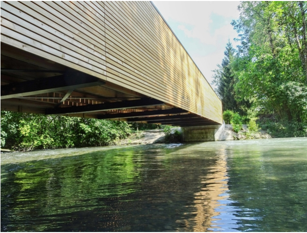
Sufficient space between the water surface and the bridge
