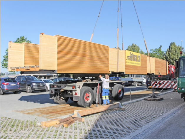
On the way: the bridge was transported in one piece
