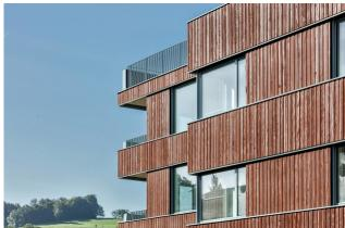
The lightweight timber facade was attached in front of the massive reinforced concrete structure. The wooden facade with sophisticated sheet metal aprons in complex geometries forms the outer shell of this superstructure.
