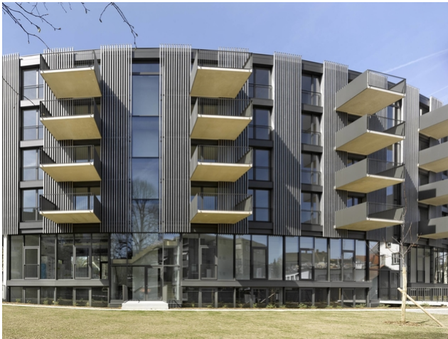
Facade view with balconies
