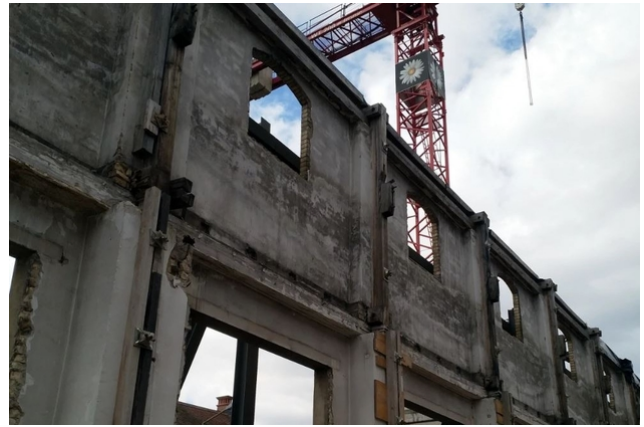
The building was deconstructed except for its facade.
