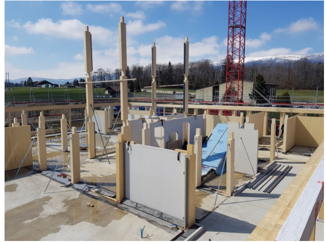
First floor under construction.
