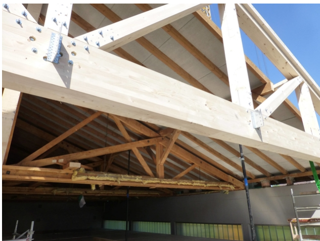
Old and new truss
