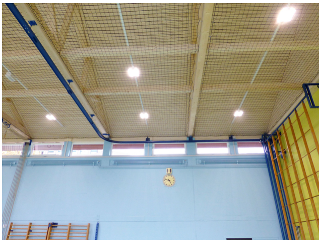
Interior view ceiling
