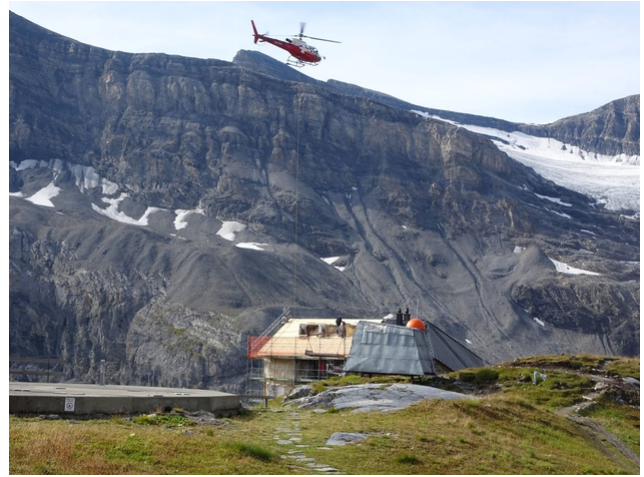
All the elements for the expansion came by helicopter.
