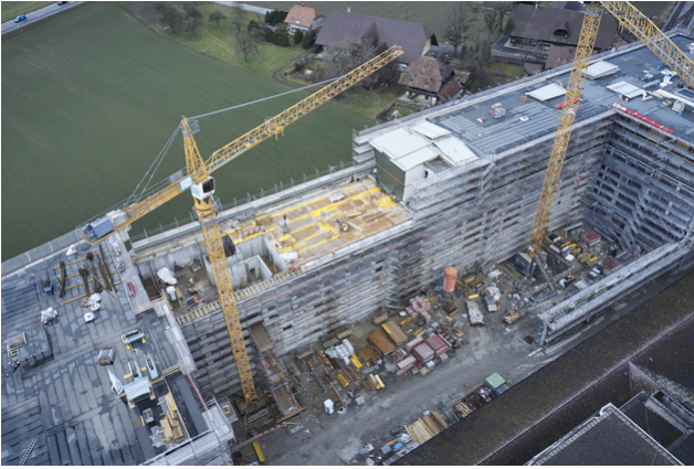
Aerial view during erection
