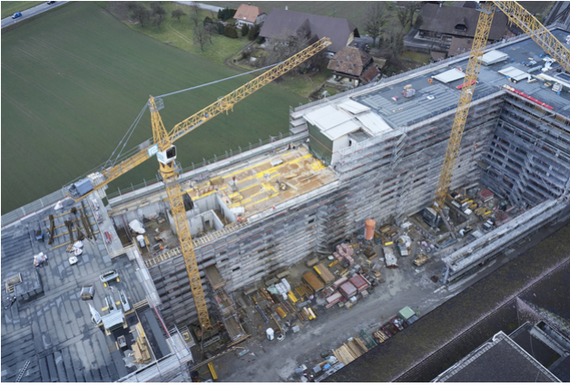
Aerial view during erection
