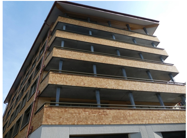
Apartment house Wolf: Covered with wooden shingles from top to bottom
