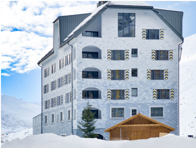
Heavy-duty roofs: Timbatec planned the roof structures
