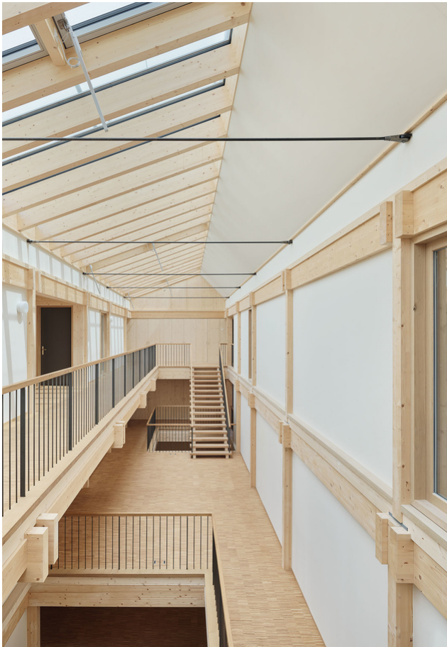
The supporting structure is made of wood except for the tie rods.
